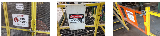
Compliant Examples of Secured Gates Requiring A Tool To Open
